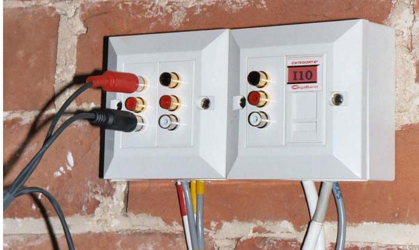
*I installed three sets of three phono sockets in the utility room roof space (each set has a composite video, right audio and left audio). The left two sets go to the kitchen and the right set (next to an RJ45 socket) goes to the lounge. Birdcam is plugged into the cabling to the kitchen, but could be plugged into the lounge sockets. (The RJ45 AVI socket will be the subject of another article!)*
